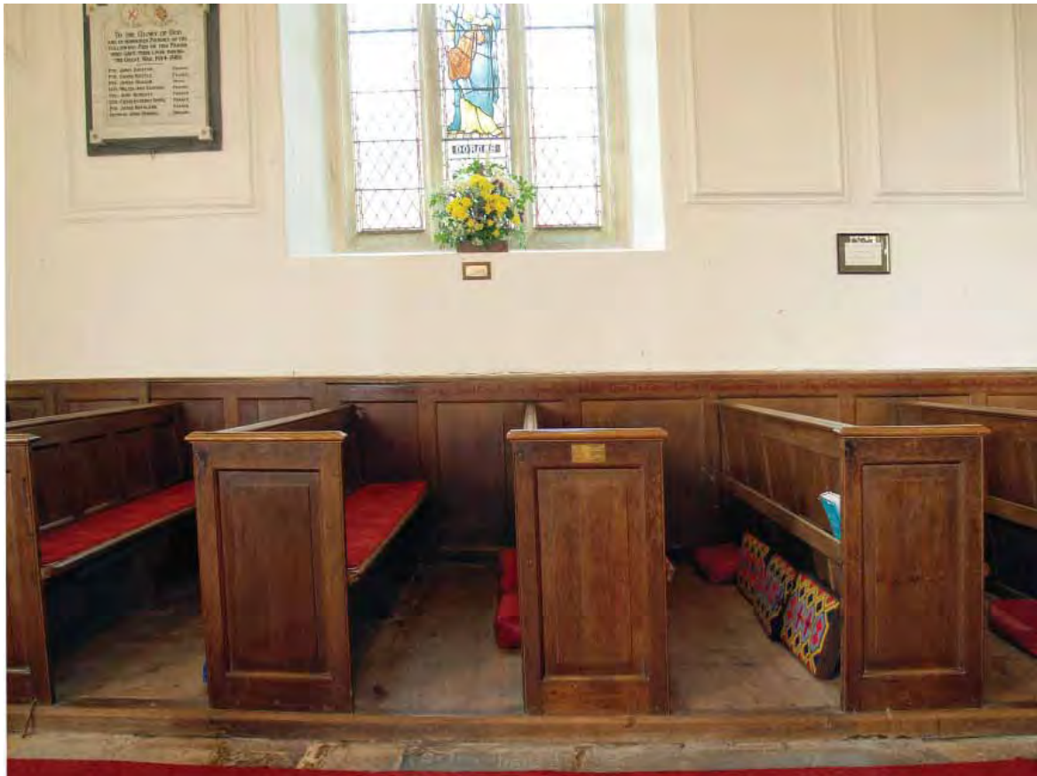
7. The box pews in the north aisle of Cruwys Morchard were completely remodelled as open benches in c.1901. However, much of the box pew fabric was recycled. The bench ends with fielded panels are part of the 1701 box pew fabric. The panelled dado was retained but reduced in height.
