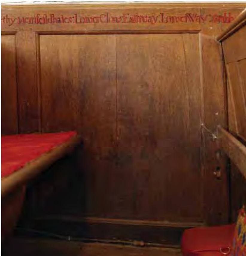
8. The wide panel of the dado against the north aisle indicates the depth, from seat back to seat back, of the 1701 box pews (29 inches, as shown on the plan). The lettering lists the names of four properties in the parish. The original box pew contained four seats for the (male) tenants of these properties.
