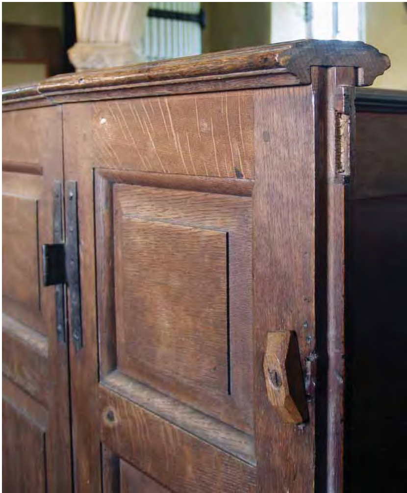
15. Detail showing the classic box pew hinge (which allows the doors to fold back and avoid obstructing the alley), a simple wooden turnbuckle for closing the door and the moulded cornice of the partition, cut at an angle to allow the door to close neatly.
